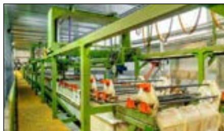
CONTINUOUS ELECTROPLATING PLANT
